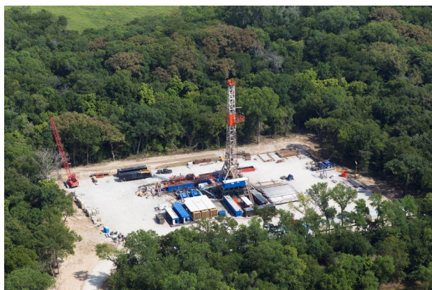
Barnett shale drilling site
